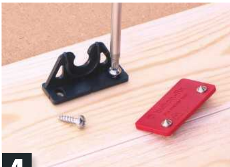
4 Remove panel and drill where points have made indents. Attach Fixes to surface with pan-head screws
